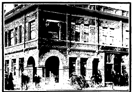
Early picture of building, built 1890.
