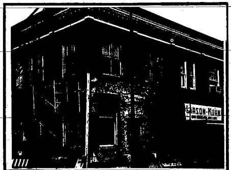
Remodeling of building, 1960.
